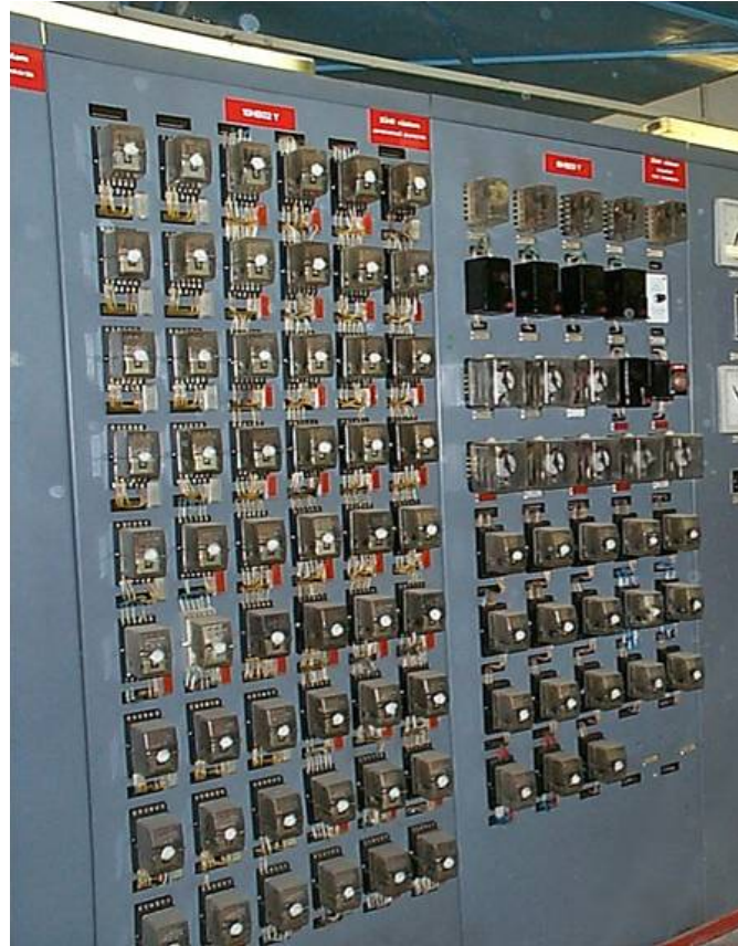
FIG. 25. Relay-based, centralized control logic.
